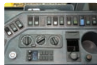
Centralized Instrument switch Panel
